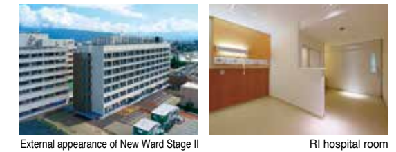
External appearance of New Ward Stage II RI hospital room
